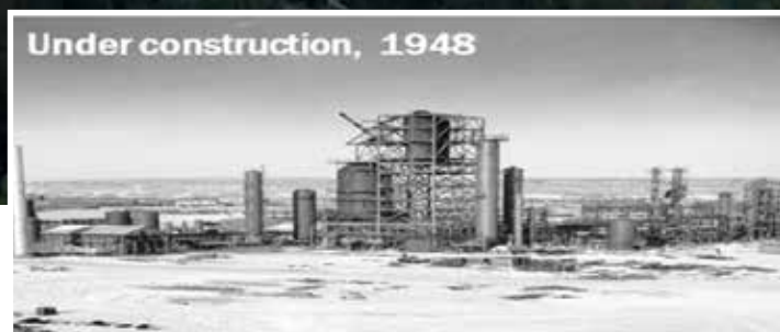
Top: The refinery's company lineage connects Billings to a deeper Western energy history. Inset: When the Billings Refinery was built in 1949, Montana and the broader Rocky Mountain region were in a time of post-war growth.
